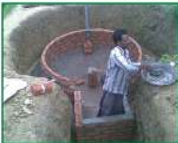
Construction of bio gas plant: alternative source of energy for domestic use
