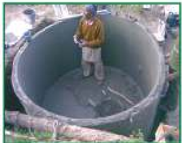
Ferro cement tank: transferring appropriate technology
